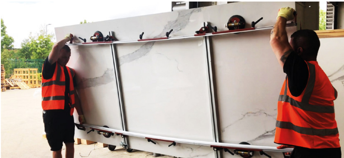
Always use handling frame to manoeuvre slabs
