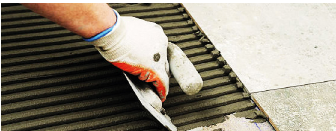
Apply adhesive in stripes running parallel with the short edge
